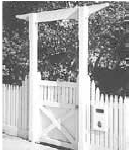
Left: A timber framed gate showing the single diagonal brace in the lower panel. Right: A 'gallows' gate with exposed double diagonal braces in the lower panel
